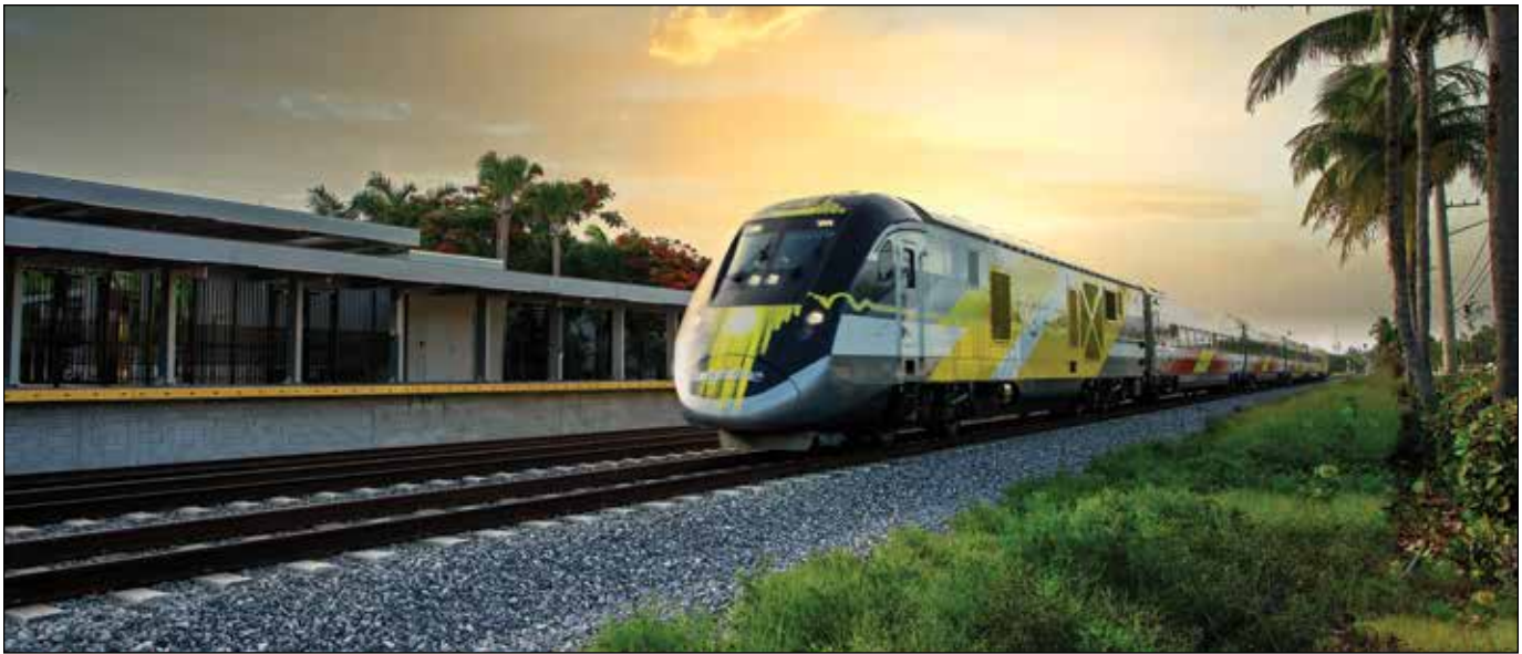
Brightline provides higher-speed rail service between Orlando and Miami, Florida while ENSCO technology continually monitors track conditions.
