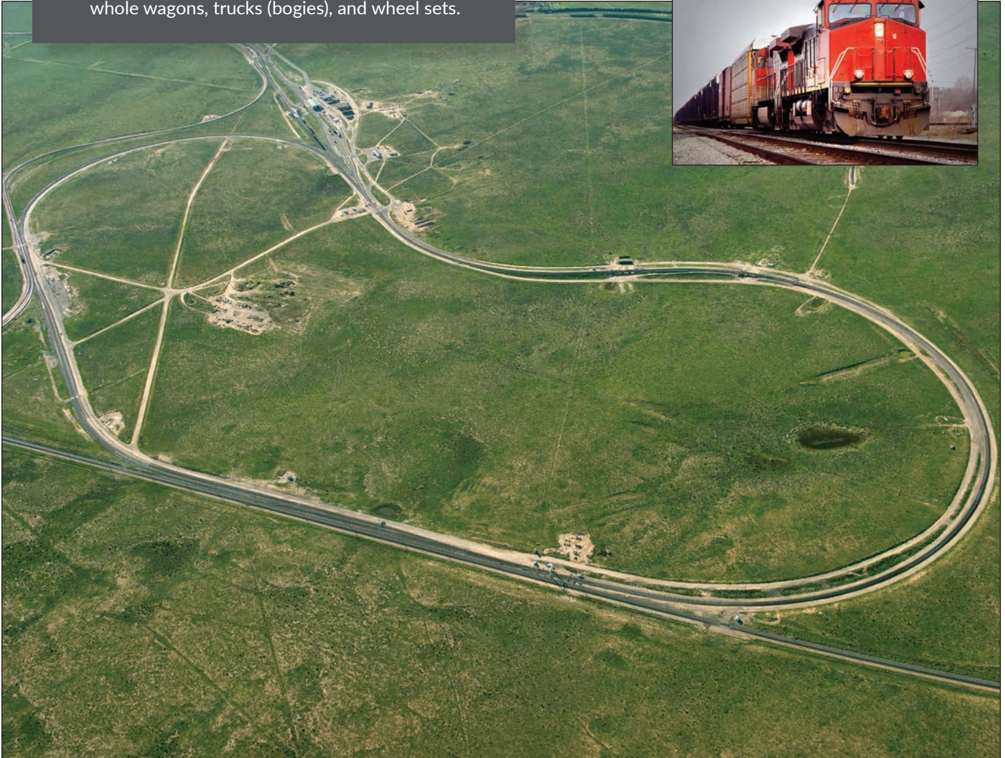
The High Tonnage Loop (HTL) at the TTC provides accelerated testing of rolling stock and track components.
